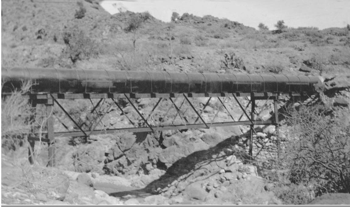
Example of steel bridge. APS Photo Library #82
