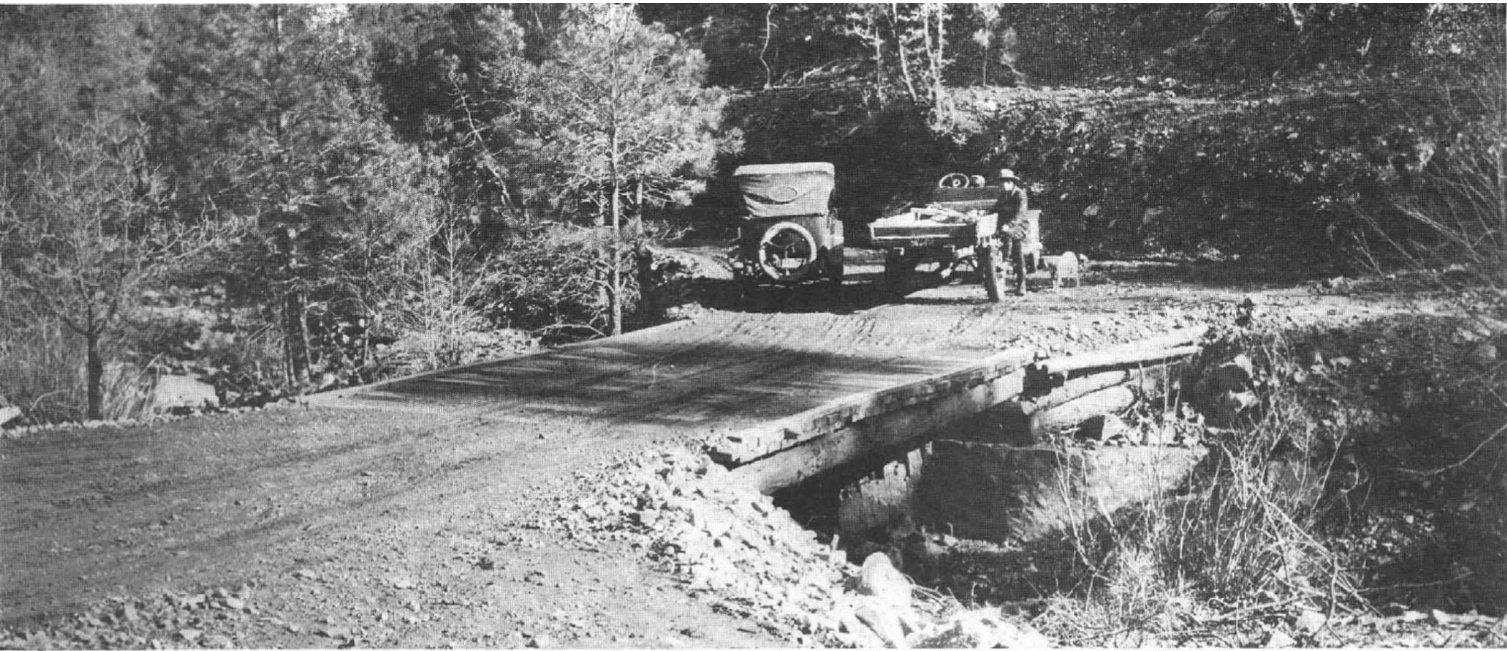
Bridge on Company road across Lynx Creek.
